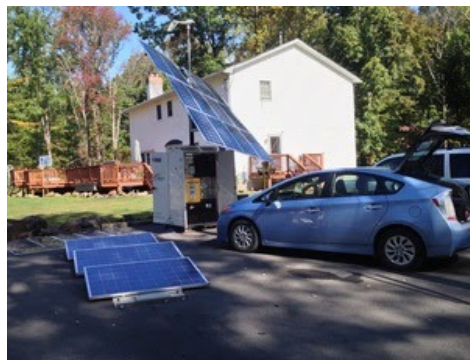
Strizki's house in the making with solar panels!
